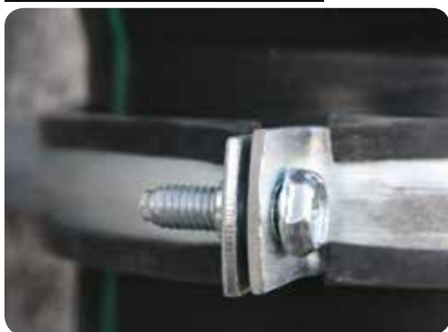
Figure 5 - Incorrect tightening:
